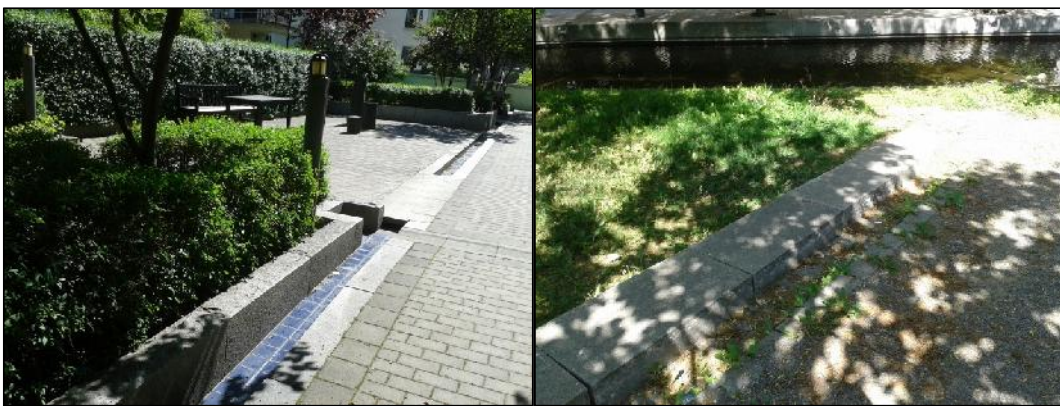
Figure 5.26: Ditches running through the residential areas which lead the storm water away (left); End-point of a ditch that opens up at the small canal in the green-avenue (right)
