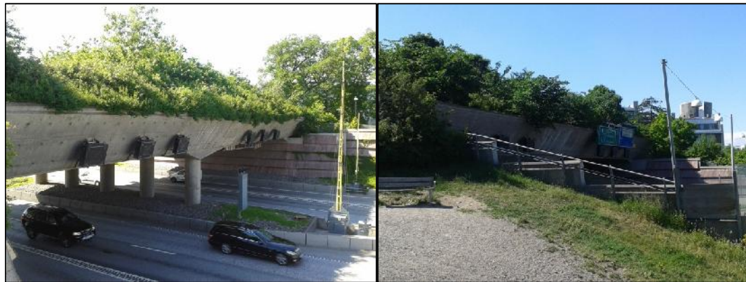
Figure 5.23: The eco-ducts over the highway which connect the Nacka nature reserve with the settlement's parks
