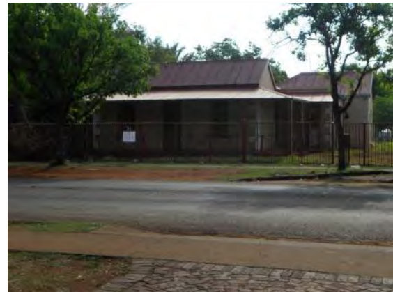
Figure 6.4 – Visual permeability of the residence from Steve Biko Avenue on the eastern border (Source: Own collection, 2013).
