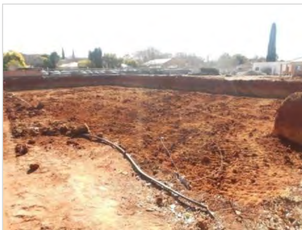
Figure 6.14 – The excavations around the Piet Malan residence (Source: Participant 4, 2013).
