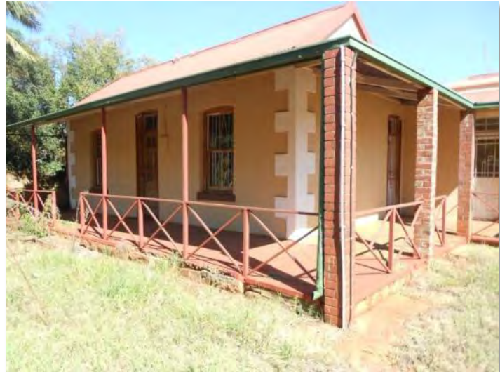
Figure 6.8 – The veranda with the stone basis and red polished surface (Source: Participant 1, 2013)
