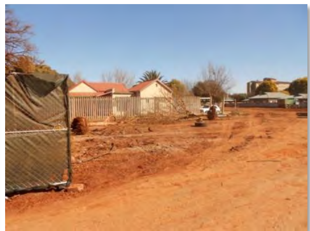
Figure 6.15 – The Piet Malan residence from the excavation site (Source: Participant 4, 2013).
