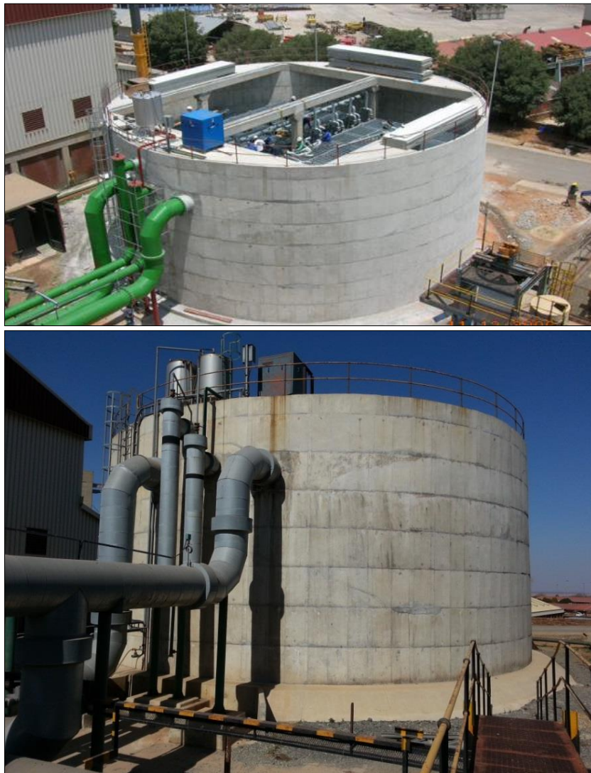
Figure 18: Ice storage dam
