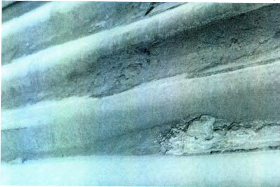
Compacted dust on roof at industrial collection site.
