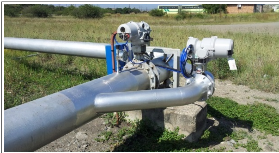
Figure 3.14: An example of a compressed air control valve[65]
