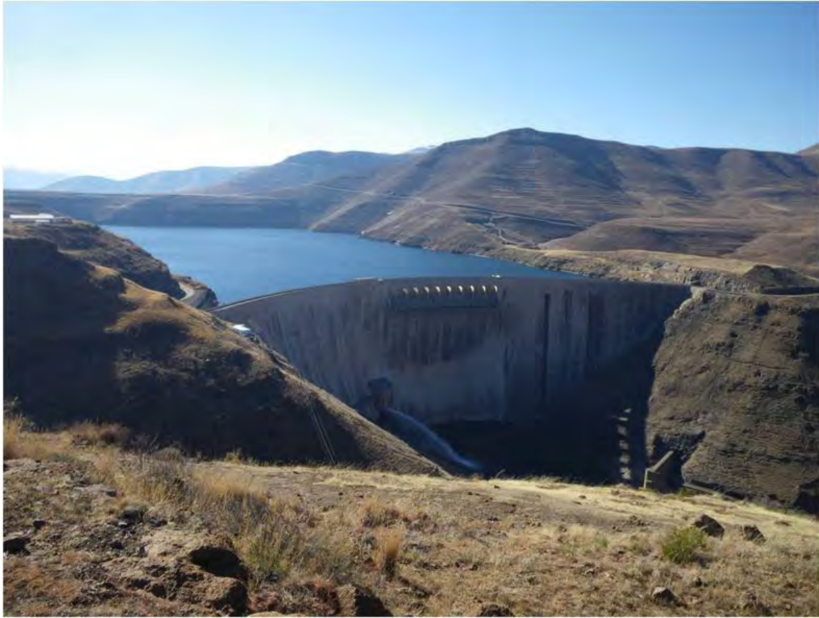
Illustration 3 The Katse Dam in Lesotho. Photograph: Martin Ginster, 2009.07.11
