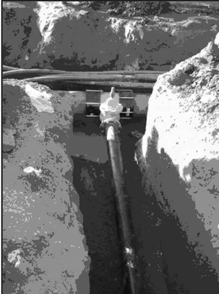
**Figure 5: Installation of missing “T-Piece” in Sebokeng**
