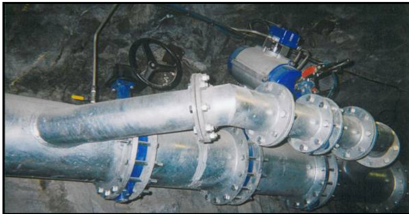
Figure 60: Control valve unit with bypass
