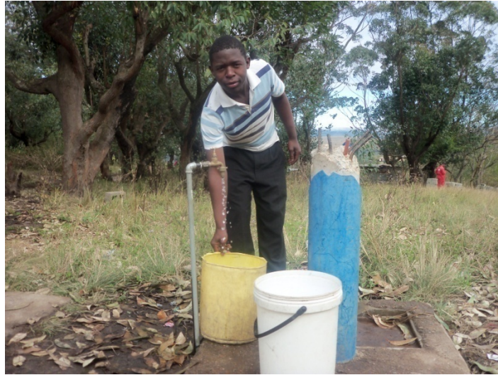
Illustration 6: Standing pipe with no pressure and the water takes an hour to fill a twenty-litre bucket in Ward 5, which resorts in the uMzumbe Local Municipality. Photographer: T. Cele
