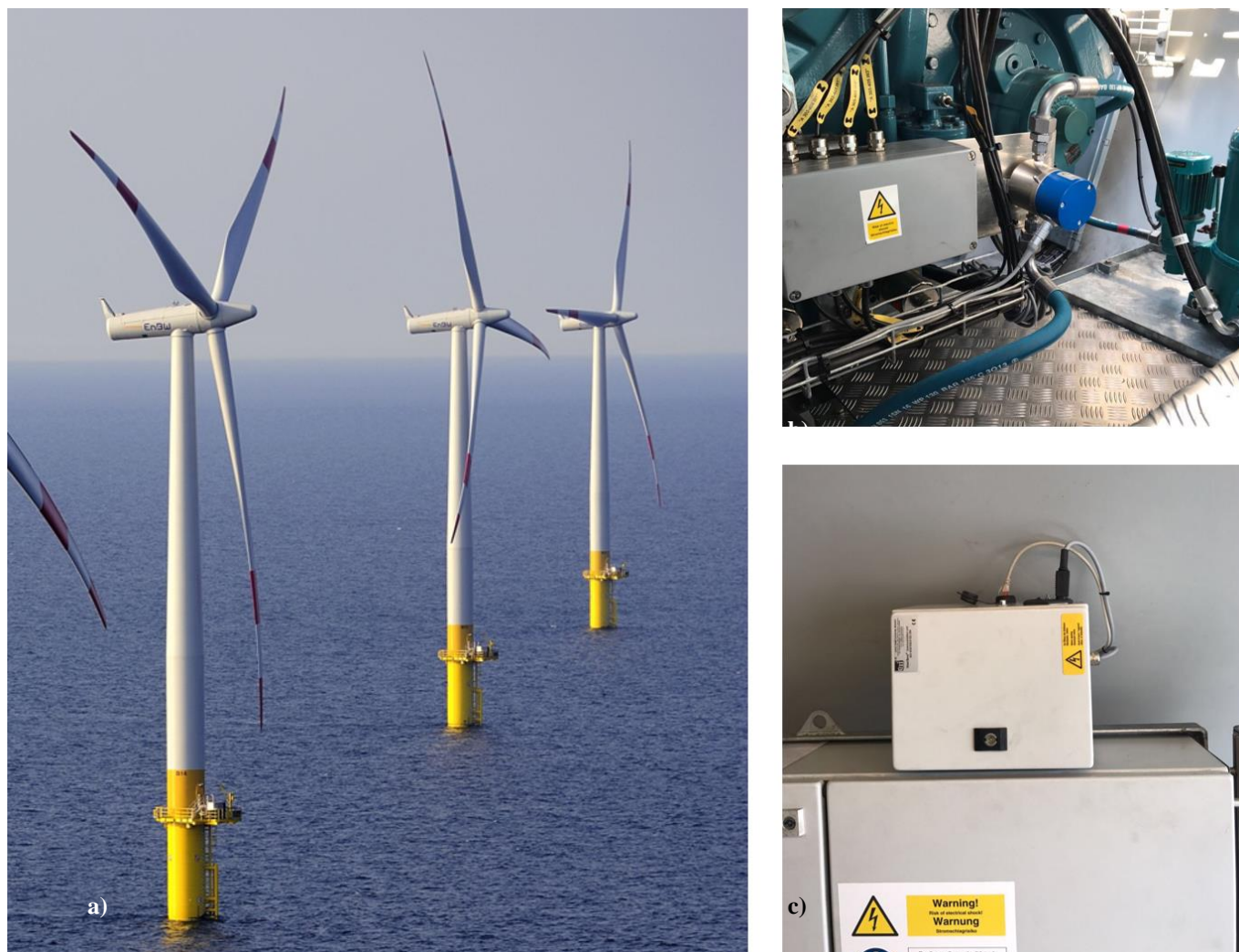
Figure 5. a) picture of the offshore wind turbine, b) WearSens ® base sensor installation in the existing cooling bypass and c) sensor communication unit.
