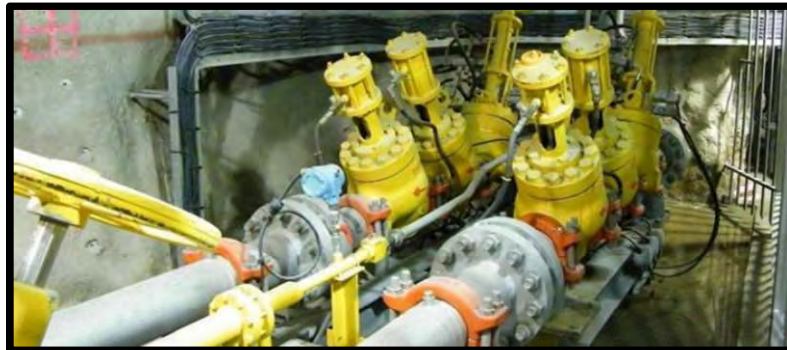
Figure 27: PRV station
