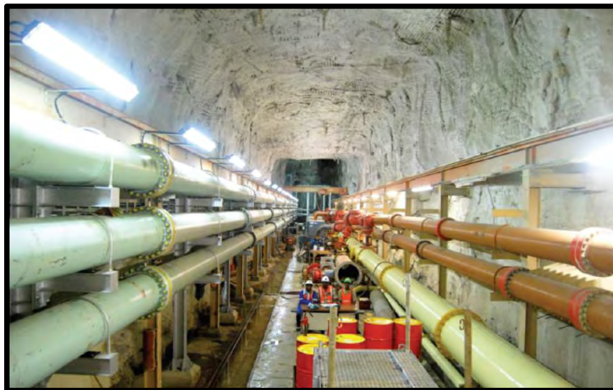
Figure 28: 3CPFS hydro-lift chamber excavated space and pipes
