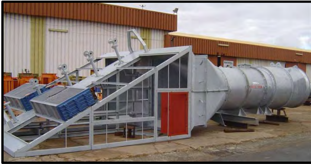
Figure 62: Construction of a CC cooling-coil HX CBAC installed on investigated mine
