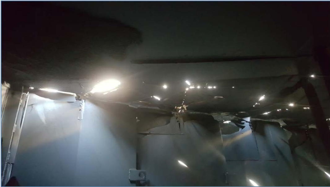
Figure 6: Power station Alpha gas pass ducting internal inspection
