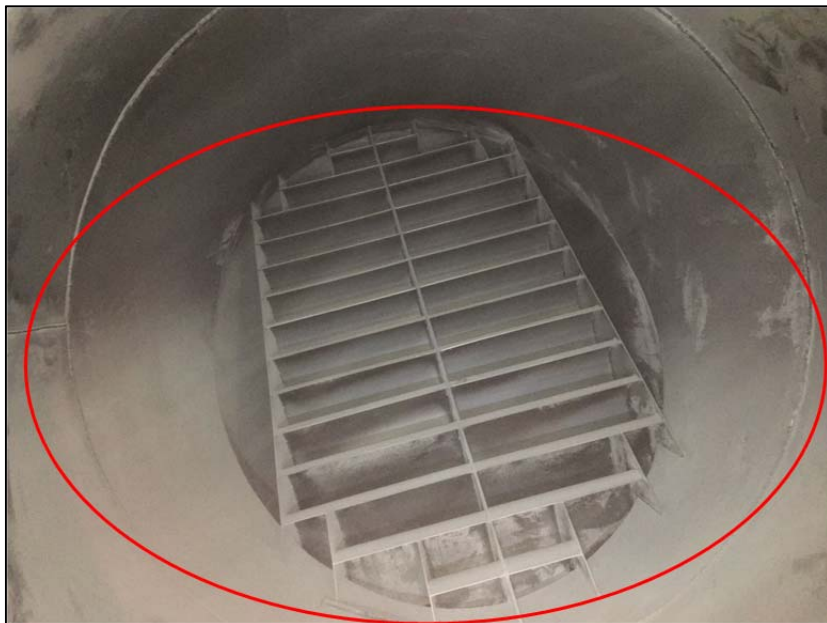
Figure 11: PA fan ducting after removal of deflector plate
