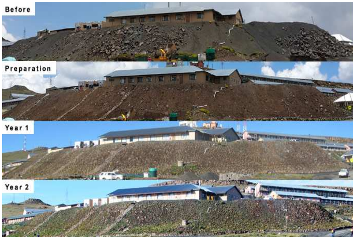
Figure 35: Establishment of vegetation on a waste rock dump and coarse tailings slope. A considerable proportion of the vegetative cover is made up by spontaneous plant species present in the soil seedbank.
