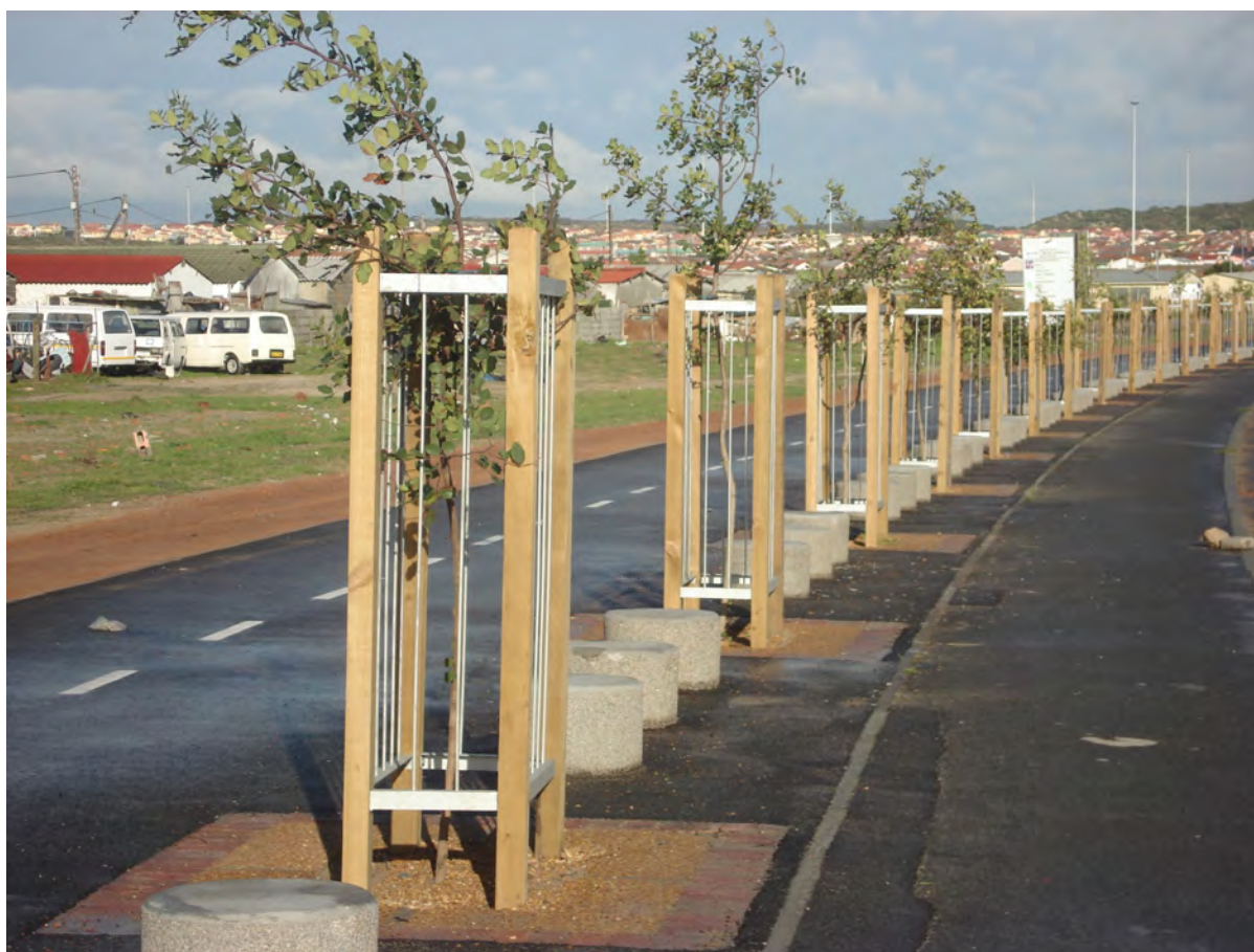
Figure 1: NMT project combining paving and tree planting in Khayelitsha
